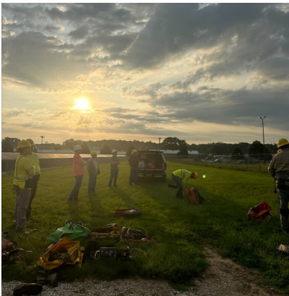
Crews preparing for early morning pole climbs.
