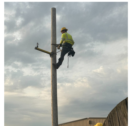
Jaxson Pauley completes his pole climb after installing a transformer gin.
